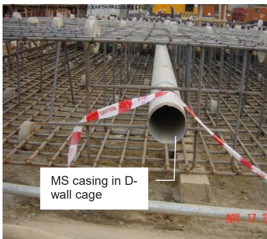
Figure 8-2 Installation of MS casing in diaphragm wall cage
