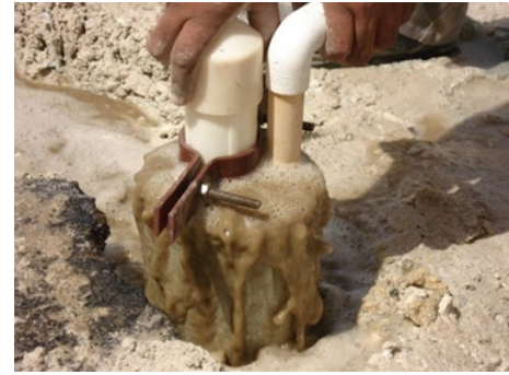
Figure 7-5 Grout overflowing (instead of water) denotes grouting is complete
