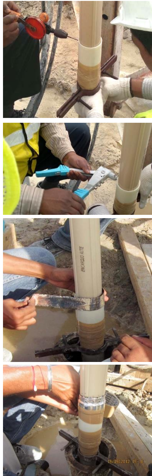
Figure 7-2 Casing installation
